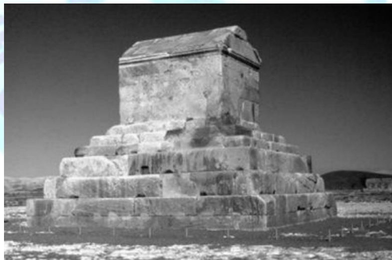
Fig 3.2: Mausoleum of Cyrus, the oldest base-isolated structure in the world
