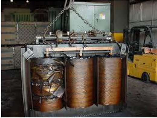
FIGURE 1: TRANSFORMER BREAKDOWN
