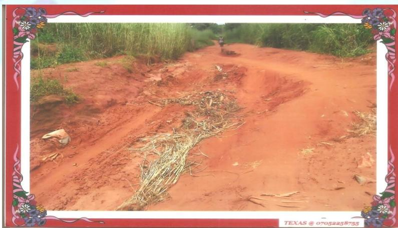
**Plate 5: Amokwu Village Square being devastated by gully erosion**
