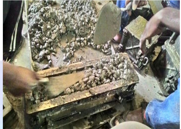
Fig. 3. Casting of beam
