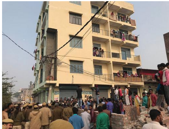
Figure 2: Illegal construction in Delhi
