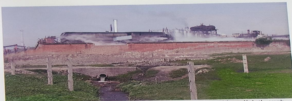
Plate 13: The effluents from Roza Sugar Factory are released in nullah through pipes.
